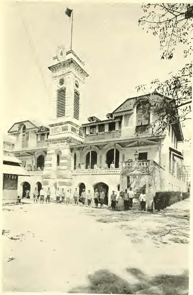
CENTRAL POST OFFICE
